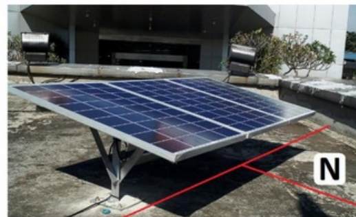
Figure-10. Solar panel arrangement.
